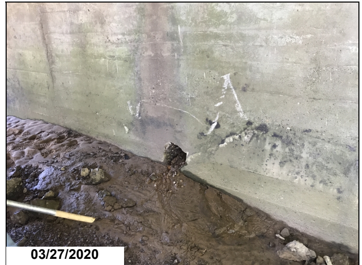
Abutment # 1-Concrete deterioration with section loss.
